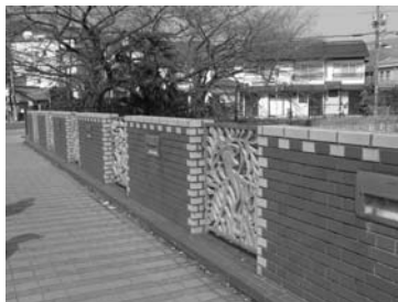
疏水に架かる橋梁
